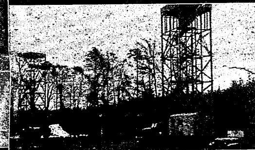
Flak Towers Loomed over the Field
