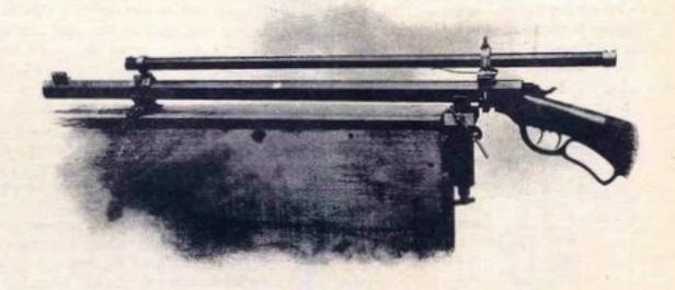
for testing purposes. More information can be derived from its use in a few hours, than can be had by ordinary rest shooting by an ordinary shooter in as many weeks, as, if at all carefully used, it has no human errors of holding and pulling. The results, therefore, are those due to rifle, ammunition and weather; the man is out of it, except so far as his loading of the rifle and judgment of wind are concerned.
